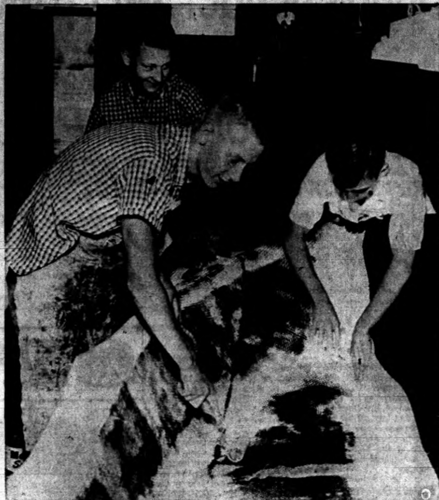
IT'S ALL FIBERGLAS — One could be riding in this proposed boat the next day after they saw it in this beginning stage at Glasto-Craft, 4811 Dixie Highway, Waterford Township. The boys are saturating one of the layers of Fiberglass with laminating resin in the mold after the color spray has been applied. They are: Denny Kind of 5825 Mill St., Waterford, rolling out the bubbles; Fred Warrick Jr., 8565 Thendara St., Clarkston, cutting the excess fiberglass off; and Jack Craven, 4560 Rockcroft, Waterford Township, placing the cloth along the bottom.
