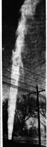
NOT SO FAITHFUL — Water gushes 150 feet into the air after an air-release valve on a 42-inch water main failed in Kansas City, Mo., yesterday. A water department foreman was injured when he was blown out of a five-foot-deep pit. He landed 20 feet away.
