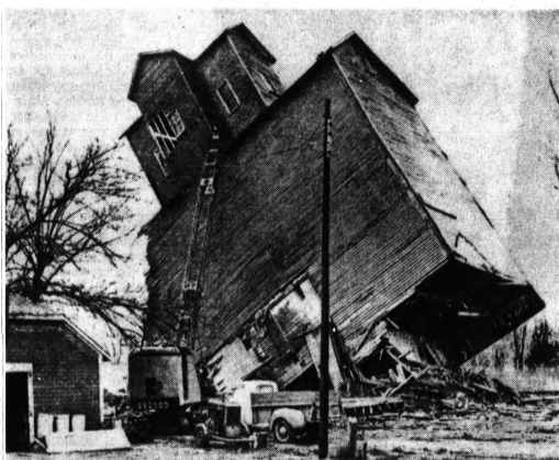
HIDDEN PROPERTY — When a construction crew went to work on the old elevator in St. Joseph, Ill., they decided to back away at it with a bulldozer. Everything went fine until the huge building
