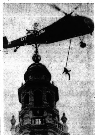
AIRLIFT FOR WORKMAN — A workman is airlifted from the tower of the Lorain University Library in Lorain, Belgium, yesterday after a cable from another helicopter broke, leaving him stranded atop the building. He had originally been lifted to the top of the tower to dismantle the ornate spire, which remains.
