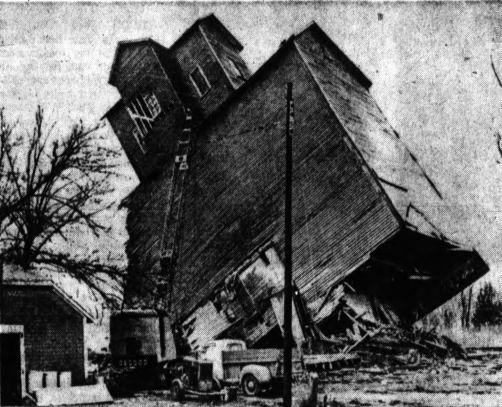
HIDDEN PROPERTY — When a construction crew went to work on this old elevator in St. Joseph, Ill., they decided to back away at it with a bulldozer. Everything went fine until the huge building tipped over and completely enclosed the machine. Now the crew is afraid to breathe on the old building, fearing it might be fatal to the valuable piece of equipment.
