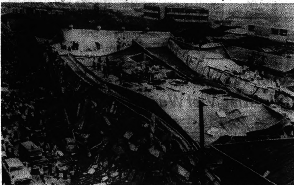
COLLAPSED BUILDING — Rescue workers scramble over a collapsed five-story apartment building in Manila today. As many as 1,000 persons were believed to be in the building when an earthquake struck the city.
