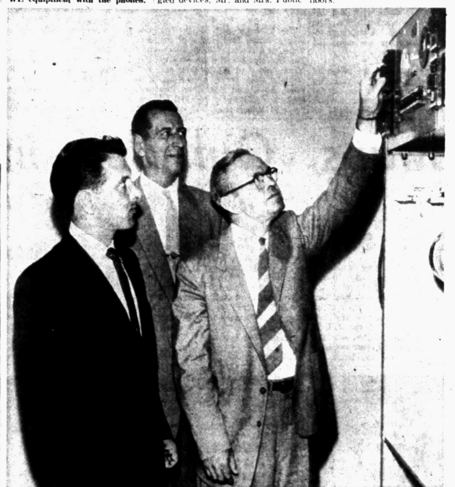
FINAL STEP — Watching as Mayor William W. Donaldson (right) plugs in the fuse activating the $50,000 telephone system at Pontiac's new City Hall are Walter Barnett (right), Michigan Bell Telephone Co. commercial representative, and Edward J. No-
