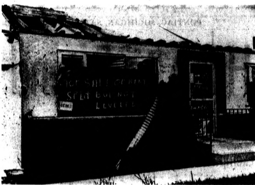
HUMOROUS HUMOR—This battered house in suburban Minneapolis was a victim of the May 6 tornadoes which hit the area. Now, the owner, Al Peterson, has put up a sign: "For sale or rent. Split but not leveled."
