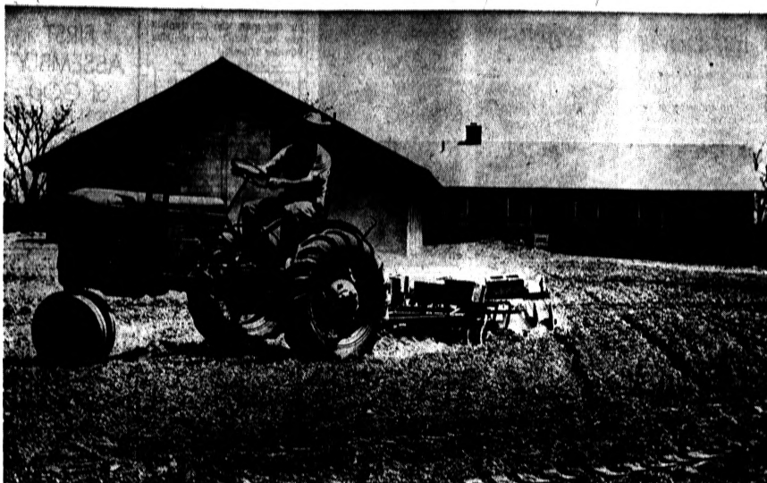
CLEARING GROUNDS AT HILLCREST BAPTIST Rev. Clarence Jackson, minister at Hillcrest Baptist Church, 1240 Doris, uses a tractor to push dirt around as he levels the ground around the new first unit. Men of the church will work with him in seeding and fertilizing the lawn area. Pastor
