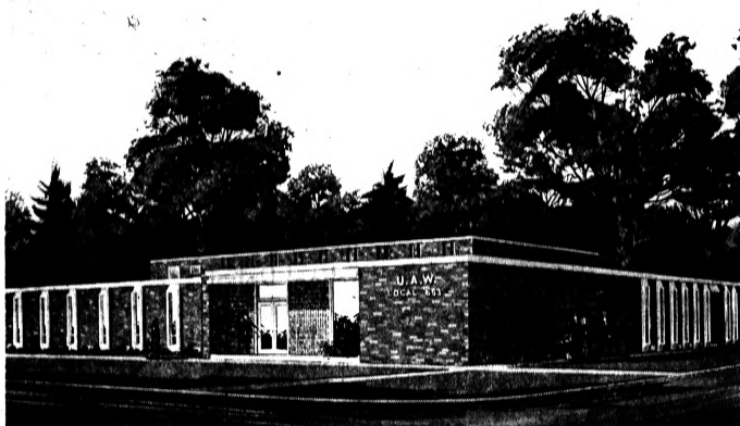
NEW LOOK — This is an artist's depiction of the future home of Pontiac Motor United Auto Workers Local 653. Now under construction at 866 Joslyn, corner of Tenyson, the $252,000 building will provide more space, more committee
