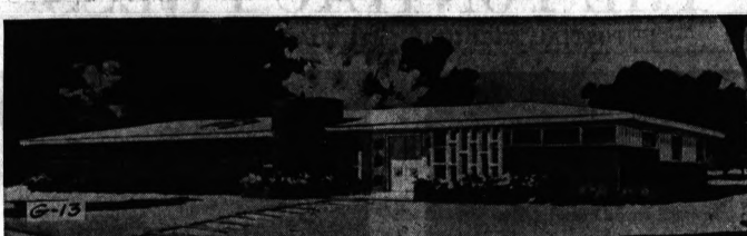
SPECIAL DESIGN — It would be difficult to pass this ranch-type house without giving it a second look. Various exterior features, including placement of windows, make it pleasingly different without excessive structural changes.
