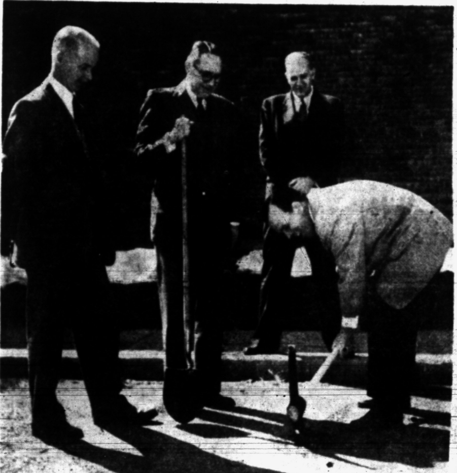
PLANETARIUM AT CRANBROOK — Officials watch the ground-breaking at the site of a planetarium building which will be added to the Cranbrook Institute of Science. To be available to school children and others at regular hours, the planetarium is the first structure at Cranbrook to be financed with publicly subscribed funds. Spokesmen say $6,000 more is needed to insure completion of the project. Watching contractor Thomas E. Killfoyle ply the pick are (left) Dr. Robert T. Hatt, director of the Institute; L. James Bulkeley, chairman of the Institute's trustees, and William E. Kapp, architect of the new annex.
