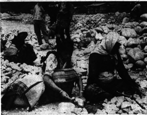
BREAKING ROCKS FOR BHUTAN'S RUNWAY — Women break up rocks for foundation of asphalt runway in Paro, Bhutan. The airfield will be the first in
