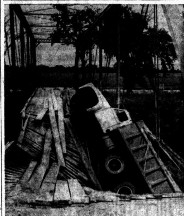
BIG SPILL —This four-ton truck, loaded with 15 tons of sand, tried to cross a 150-foot bridge over the Smoky Hill River near Salina, Kan. It didn't make it. The bridge fell in. So did the truck. Here owner-driver Roger Cline, unhurt, surveys the plight of his eight-week-old vehicle.
