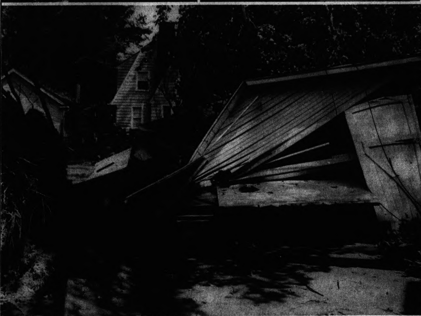
The most destructive storm in the history of Detroit Edison
