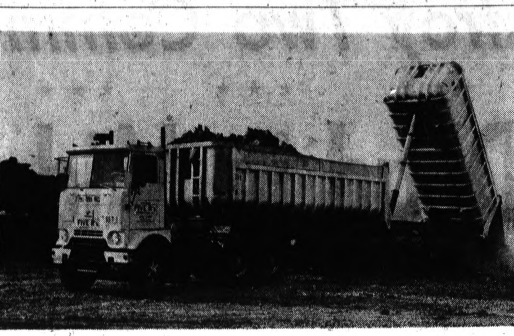
BIG RIG —One of the GMC Truck & Coach Division rigs operated by Five R's Construction Co. of Drayton Plains, dumps a load of clay hauled to a dumping site from the Chrysler Expressway project. Each rig hauls 57½ tons of earth. The firm's modern fleet is revolutionizing the aggregate and earth moving industry in Michigan.
