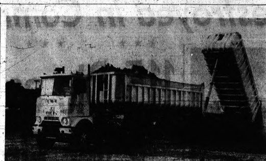
BIG RIG—One of the GMC Truck & Coach Division rigs operated by Five R's Construction Co. of Drayton Plains, dumps a load of clay hauled to a dumping site from the Chrysler Expressway project. Each rig hauls 37½ tons of earth. The firm's modern fleet is revolutionizing the aggregate and earth moving industry in Michigan.
