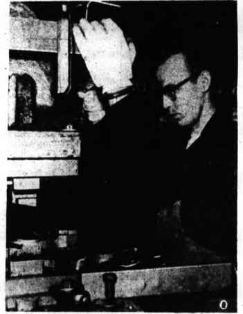
SMALL PRESS OPERATOR — John Edwards, 3062 Adams St., uses a small press to flange (make a projecting rim or edge) grill supports. Edwards says he flanges about 1,500 pieces a day.
