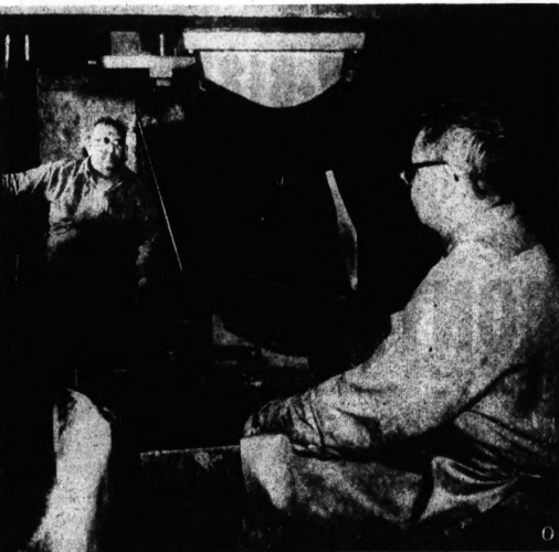
DROP HAMMER OPERATORS — These two men make sections of roofing panels for buses. The drop hammer shapes flat pieces of metal into ordered specifications. J. C. Jones, 132 Mt. Clemens St., holds the sheet of metal in place while Erick Bearson, 533 N. Perry St., drops the huge hammer.
