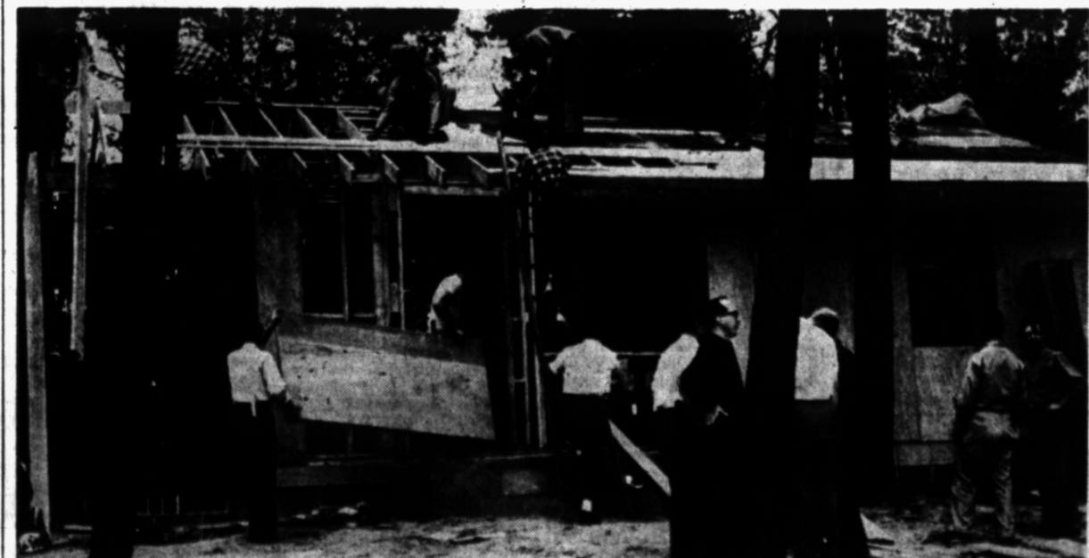
BUILDING BEE — Part of the 80 DeVlieg Machine Co. employees who joined in a building bee Saturday at Camp Oakland are shown as they rush construction of a 38 x 18-foot cabin which will house groups of children for two week summer vacations. Employees of the Ferndale company started work at 5 a.m. and hoped to finish by dark but rain delayed completion of the project. The volunteer workers, who supplied all their own construction materials, said they would finish the job next Saturday. Camp Oakland on E. Drahner road about one mile south of Oxford is under the jurisdiction of Oakland County Juvenile Court.
