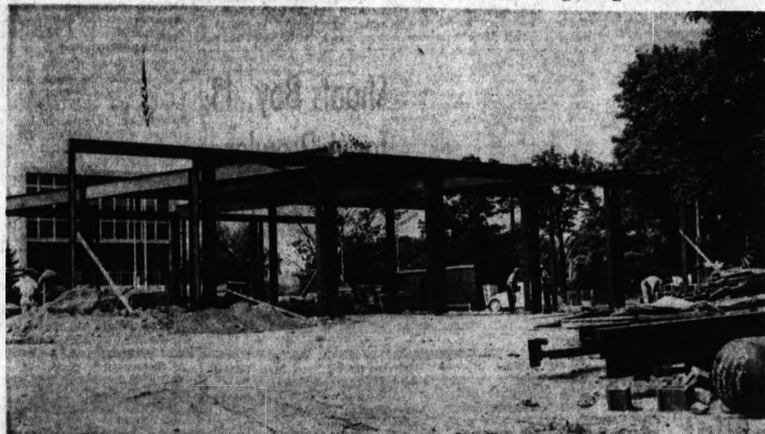
FIRE HALL GOING UP —Steel workers have erected beams at the site of the future Civic Center fire hall across East Pike Street from the Public Safety Building. One of several city projects contributing to payrolls in Pontiac this summer, the fire hall is to be completed by the end of the year. The total bill, including construction and furnishings, is to be around $75,000.
