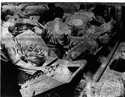
BELT WITH A BRAIN—A conveyor belt with a magnetized "brain" is helping to cope with the Christmas rush at the airport facility of the post office at San Francisco International Airport. Here sacks of mail are ripped onto the belt by the press of a button. Workers called coders receive telephone instructions from dispatchers on where each sack should go. They induce a magnetic destination code into the belt under the sack. When it reaches its destination, the sack is automatically shoved off to one of five airline docks.
