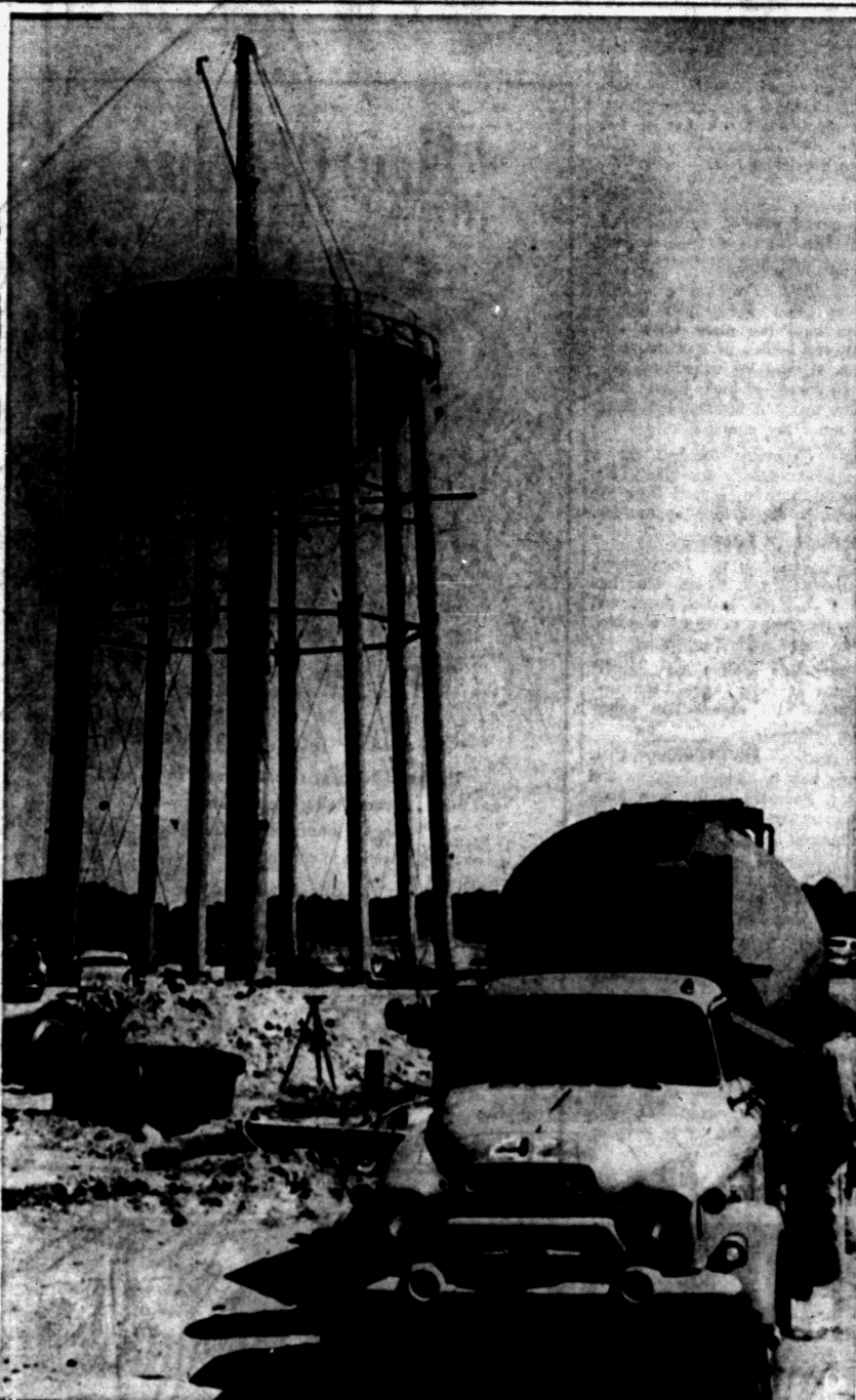
500,000 GALLON TANK—The huge tank shown under construction will have a capacity of 500,000 gallons and will rise 120 feet above ground at the Army Ordnance warehouse being built just off East
