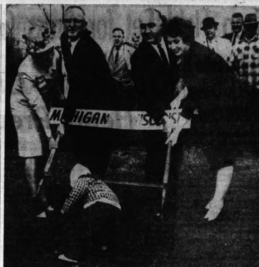
AN UNINTERESTED SPECTATOR — Two-year-old Melissa Cavosie of Hurley, Wis., was only interested in the digging when she walked into the picture during ground-breaking ceremonies at Ironwood for twin bridges that will carry U.S. 2 over the Montreal River at Ironwood and Hurley, Wis. Doing honors at the ground breaking were (from left) Sharon Hautanen who is Miss Ironwood; Michigan State Highway Department assistant chief bridge engineer Joe Orvace; Wisconsin State Highway Department Chairman Harvey J. Grasse and Jaumeen Kessler who is Miss Hurley.
