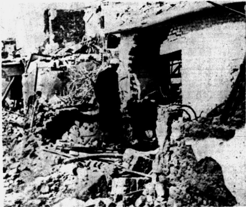
BOMBING RUBBLE — A lone Egyptian inspects the ruins of houses at Helopolis, a suburb of Cairo, after they were struck by bombs from Anglo-French planes that missed their objective, the nearby Almaza military airfield. According to Cairo sources, the homes are those of employees of the Helopolis Metro Co., several of whose trolley cars were also hit by the bombs.
