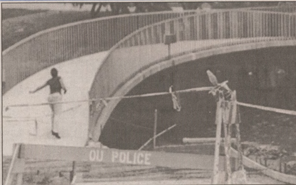
Detour: Students traveling to and from residence halls have to figure out alternate routes due to construction zones.
