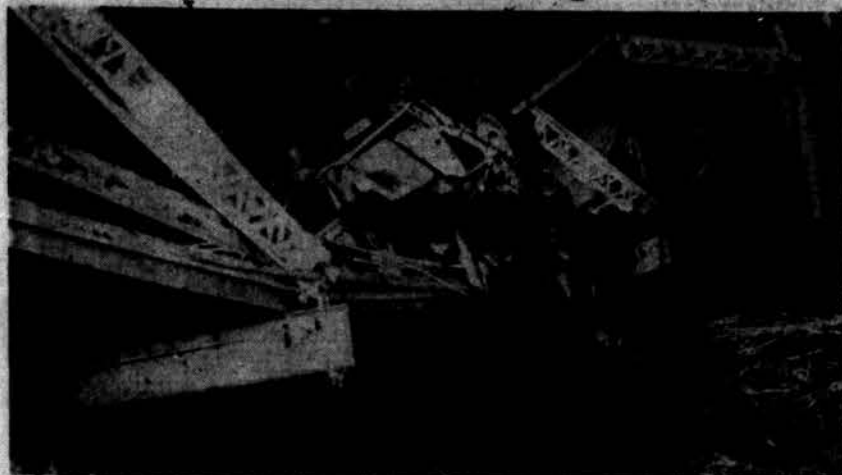
BRIDGE KNOCKED OUT —An automobile was wrapped around the steel girders of a bridge near Colfax, Wis., last night when a tornado struck the west-central Wisconsin area. The car was bent double.
