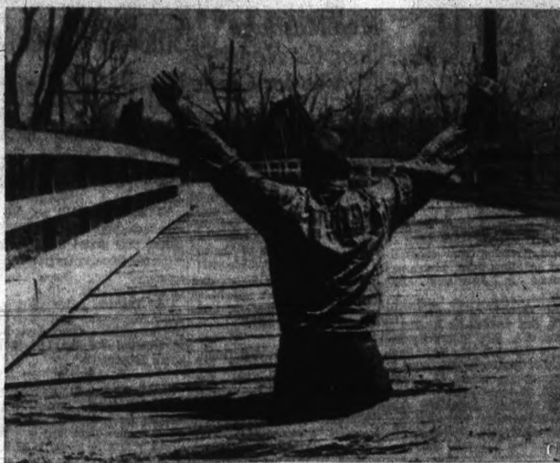
HE PROVED HIS POINT — A 200-pound man stands in a hole in the wooden plank of a bridge at Lincoln, R. I., to demonstrate the unsafe condition of the span. John T. Russell, a local photographer, said he tried for weeks to get town officials to order repair of the bridge.
