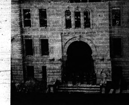
Courthouse Under Construction—1902-05
