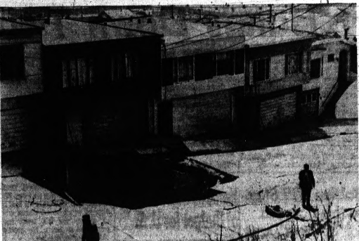
FIRE CAUSES HOLE — A fire which has been burning in a railroad tunnel which runs under San Francisco's Proterio Hill district since Saturday caused Missouri Street to cave in yesterday and threaten these new homes with destruction. The tunnel runs under those of at least 25 other homes built on top of the tunnel.
