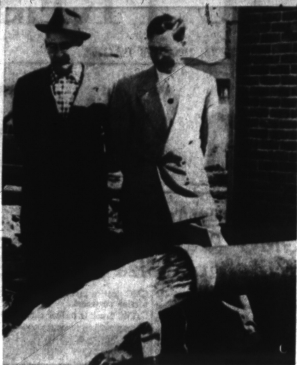
COOL AND CLEAR—Water Dept. Superintendent Joseph B. Gable and Harold A. Kelly, of water engineering consultants Jones, Henry and Williams, of Toledo, watch as water gushes from a new well in Beaudette Park. The well, expected to be hooked into the municipal water system this week, is capable of producing more than 2,000,000 gallons a day. Powering the pumps is a 150 horsepower engine, largest used on any city well. Officials say three new wells like this one every year are essential to keeping pace with city water needs.
