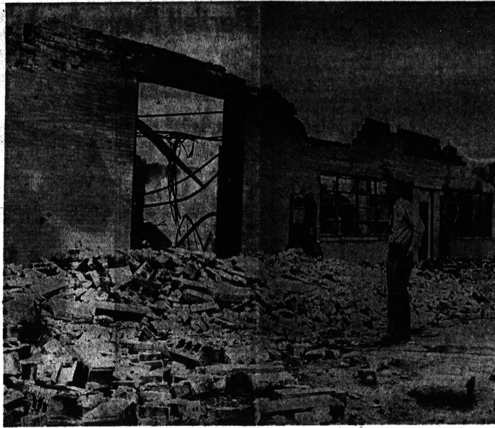
Investigates Plant Fire — Looking through the rubble and charred remains of the Fabritec, Inc. plastics plant in Lapeer is Police Chief Matthew Dougherty. Police and fire officials have been unable to discover the cause of the $500,000 blaze which destroyed the plant. Only portions of brick and concrete walls were left standing after the fire swept through the building and touched off several explosions inside the plant early yesterday morning.
