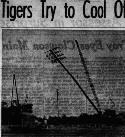
GOING UP — Workers start holding the first light pole in position at Jayco Park as the project to give the city of Pontiac its first lighted baseball field gets under way. All the area is expected to be in their proper place and ready for duty very soon.
