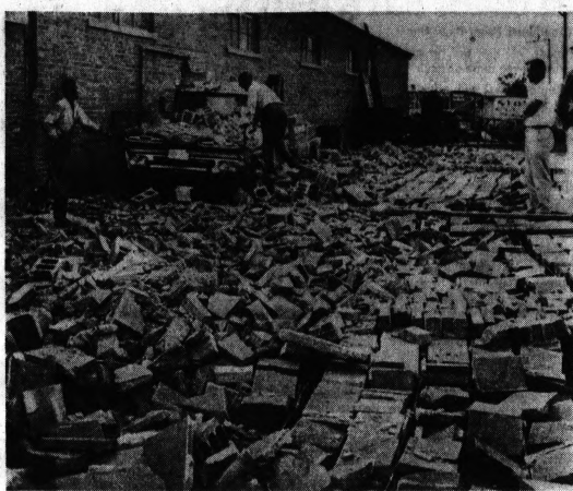
WIND DAMAGE —When tornado-like winds hit a brick-wall addition to a Chicago factory early today, the wall toppled into an alley and made the alley appear to have been brick-paved. Largest pile in the brick pattern came where they hit and covered a parked truck.
