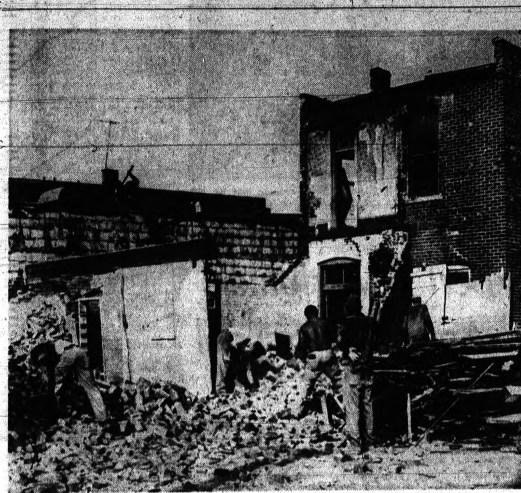
DEMOLITION PROJECT —As part of the renovation of the old Behm's Dairy building, 311 Main St., Rochester, the rear section of the two-story structure is being razed. The front portion will be extensively remodeled before a new business, Welch's Downtown Gift Shop, goes in there later this year.
