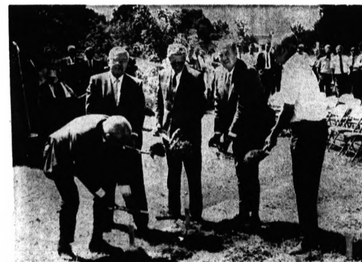
DIRT IS DUG—A group of county officials turned token shovels of earth last week to mark the beginning of construction for the new $2-million county service building to be located on Watkins Lake Road north of Pontiac Lake Road. The facility will house the Department of Public Works, Drain Commission and other functions. Breaking ground
