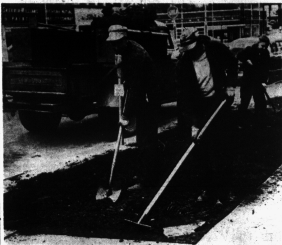
CLEAN-UP WEEK PROJECT — A Detroit Edison Co. maintenance crew is shown resodding a plot in front of offices at 58 W. Huron St. Left to right are Wayne Lehto, of 4831 Maycrest, Waterford Township, and Howard Schultz, of 2850 Lapeer Rd., Lake Orion.
