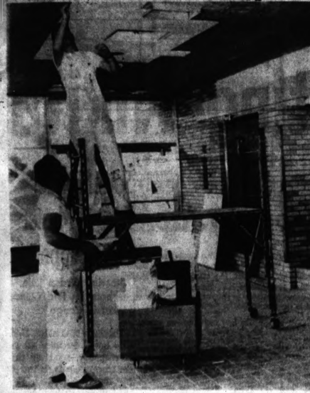
FINISHING THE TICKET OFFICE — Workmen rapidly near completion of the ticket office in the Pontiac Municipal airport terminal. It's at the counter above that you'll be buying tickets when the first commercial airline service begins at the airport in a month or so. The terminal also has a waiting room, dining room and offices.
