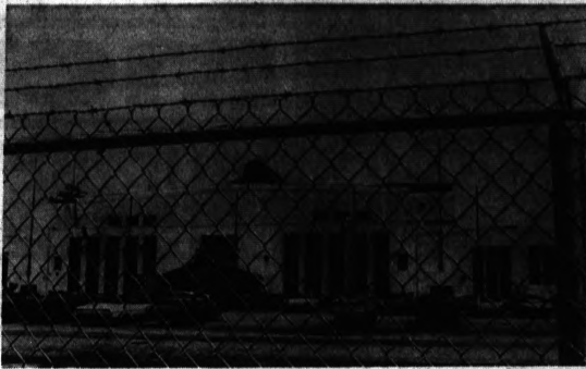
SECURITY PRECAUTION — A chain-link fence with a barbed-wire top protects the western perimeter of the International Amphitheatre in Chicago. The fence was
