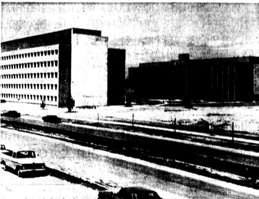
NEW MSU BUILDINGS — Michigan State University will dedicate its new $5.2 million biochemistry building (left) and its $6.6 million chemistry building June 3-5. MSU officials said the two new buildings contain some of the most complete, most modern facilities available anywhere for teaching and research.
