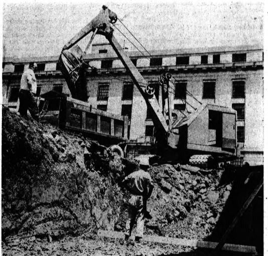
WORK BEGINS—Ground was broken yesterday on addition to The Pontiac Press building, 48 W. Huron. The 18,000-square-foot wing will house seven new press units capable of
