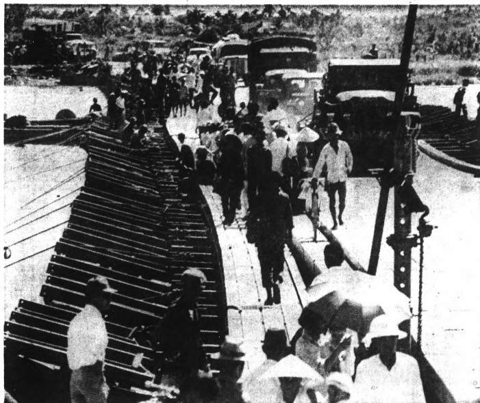
BRIDGING SAIGON WITH MEKONG DELTA —Civilian and military traffic flows across a pontoon bridge constructed by U.S. and Vietnamese engineers to span the Vaico Oriental River, a tributary of the Saigon River, at Ben
