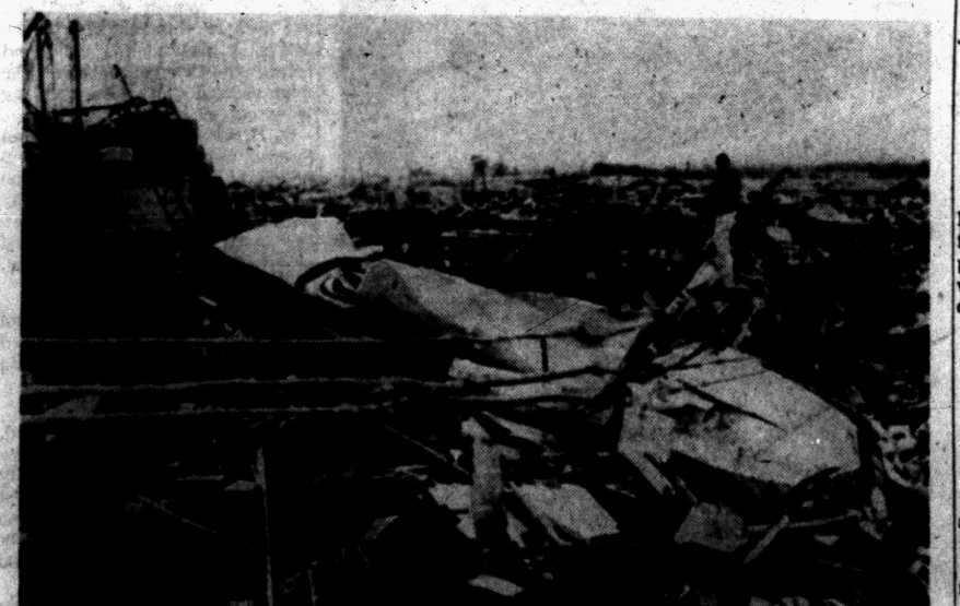
THERE WERE HOMES — A lone spectator looks over the splintered wreckage of a residential section of Rusk Heights, Kansas City suburb. In left foreground are ruins of part of a school. Beyond is wreckage of homes after twister struck.
