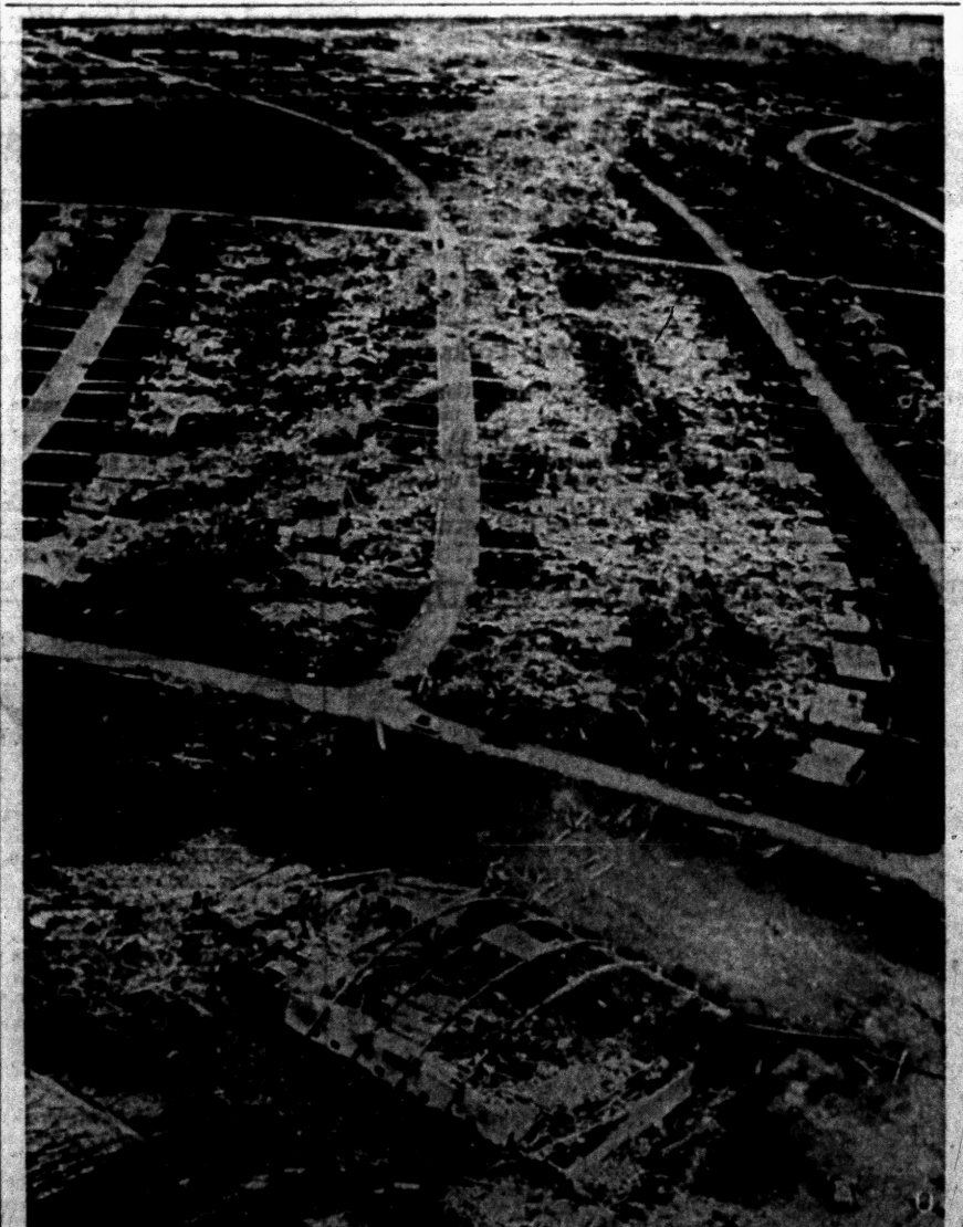
PATH OF TWISTER — This low aerial view shows the devastating path of last night's tornado through the suburban Heights residential area in Kansas City. In the foreground are ruins of a church.
