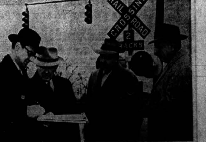
OFFICIALS INSPECT CROSSING — Officials of the State Highway Dept., Public Service Commission, Grand Trunk Western Railroad, and the city inspect the railroad crossing at South Saginaw street and Wilson avenue. The Commission ordered the installation of safety gates at the crossing earlier this year. As the Highway Dept. was not consulted then, yesterday's meeting was called, according to Theodore M. Vanderstempel (second from left), Pontiac traffic engineer. From left to right are D. W. Hughes, railroad safety inspector for the Commission, Vanderstempel, R. W. McClish, and Palmer Slack, engineers for the Highway Dept.
