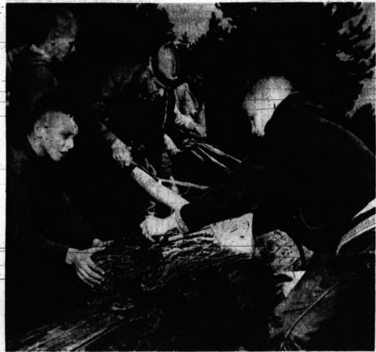
WORK CREW — Stripping bark off locust poles is just one of the chores Boy Scouts tackled at Proud Lake State Recreation Area Saturday. Armed with shovels, rakes, paint brushes and the like, approximately 1,150 scouts from the Redford District helped to get the area in shape for Memorial Day. The scouts, who camped in tents for their work bee, were earning credit for their merit badges and having a good time too.
