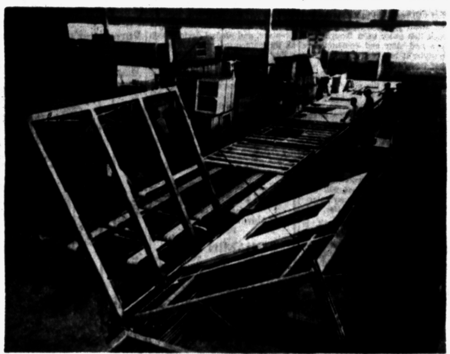
ASSEMBLY LINE PRODUCTION—Homes, too, said the Price Bros. of National Homes Corporation, should be mass-produced by assembly line technique. The above photo was taken in the Lafayette, Ind. plant where a complete side panel moves smoothly from original jig to loading dock, all in a matter of minutes. The swivel table turns
