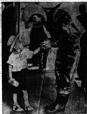
SHE'S A MODEL —That's no spaceman, Danny. It's model Meredith Proctor. She wears a suit designed for use in fueling missiles and in other such toxic areas. It contains its own oxygen supply and an air condition system and was displayed at the opening session of the annual Association of the United States Army meeting in Washington. Danny? He's 3-year-old Danny Darling of Darling, Pa.
