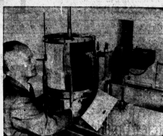
MODERN GUTENBERG — Refugee Chinese scholar Chung Shu Kwei shows his invention in Washington, D. C., which, he says, could provide inexpensive printed material for millions of Chinese for the first time in history. The photo typesetter consists of a translucent drum, 7,500 Chinese characters and a 35mm camera. Operator rotates the drum until the proper character is in front of the shutter. Film strips are pasted together to make full pages, then photographed and printed.
