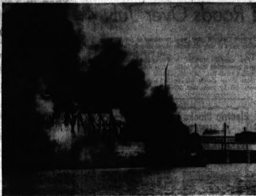
FIRE ON THE POTOMAC — Smoke billows from blazing wood pilings on the railroad bridge across the Potomac River into Washington yesterday during a fire which halted rail traffic on the main north-south rail route on the East Coast. The span is the only one crossing the river within 50 miles. Partially visible in the background are the Washington Monument and the Jefferson Memorial (right).
