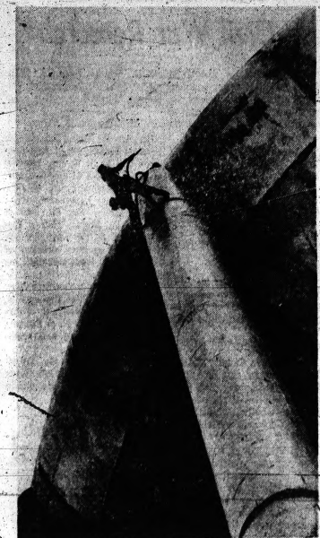
MAN IN SPACE — Dangling high atop the new 3-million-gallon elevated water tank at Edison and Montclair, this worker appears to be watering the water tank. Actually, he's hosing it down with a gleaming coat of silver paint. The tower is almost ready to hold the Detroit water scheduled for arrival July 1.
