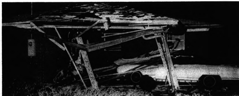
DYNAMITE DAMAGE —An early morning dynamite blast shattered the roof and carport yesterday at the
