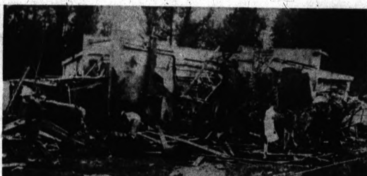
PROBE WRECKAGE — Rescue workers probe the wreckage of a reinforced concrete building in the naval propellant plant at Indian Head, Md., where five civilians, the entire crew working in the building at the time, were killed in an explosion Friday night. A Navy spokesman said research in the manufacture of rocket fuel was being conducted in the building. It was the third accident at the plant this year.
