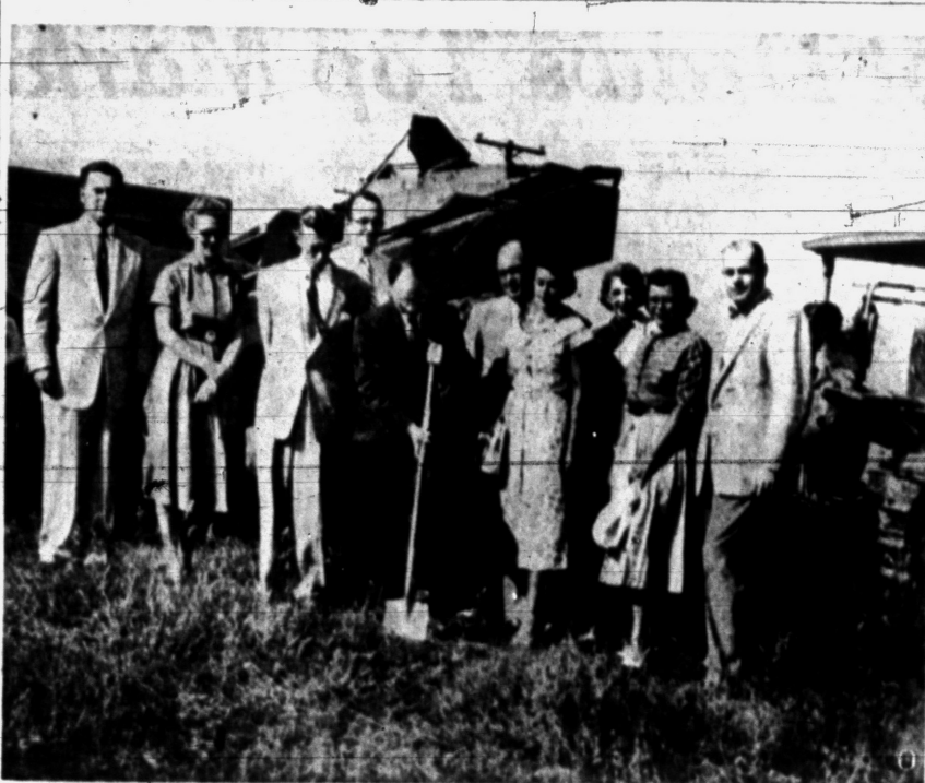
SPADE WORK —Turning one of the first spadeful's of earth for the new North Hill Elementary School yesterday is Board of Education secretary Lewis Arscott, who followed board president L. G. Harding in the ceremonial rite. Excavation for the new buildings will get under way in the near future.
