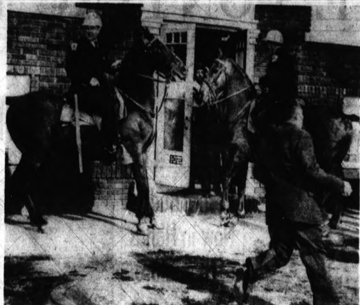
CLEVELAND VIOLENCE — Mounted police confront spectators near where a demonstrator minister was crushed under a giant earth mover yesterday. His death sparked further violence, as demonstrating mobs at the Cleveland school construction site hurled bricks and bottles at police, and beat the operator of the earth mover.
