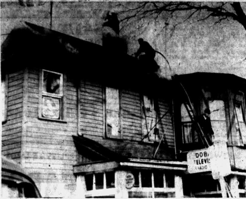
ROCHESTER FIRE QUENCHED — Firemen and volunteers extinguished a fire in Rosso apartment and store building in Rochester yesterday afternoon. The structure, one of Rochester's oldest, is located at Main and 5th streets. Damage was held to an estimated $7,000.
