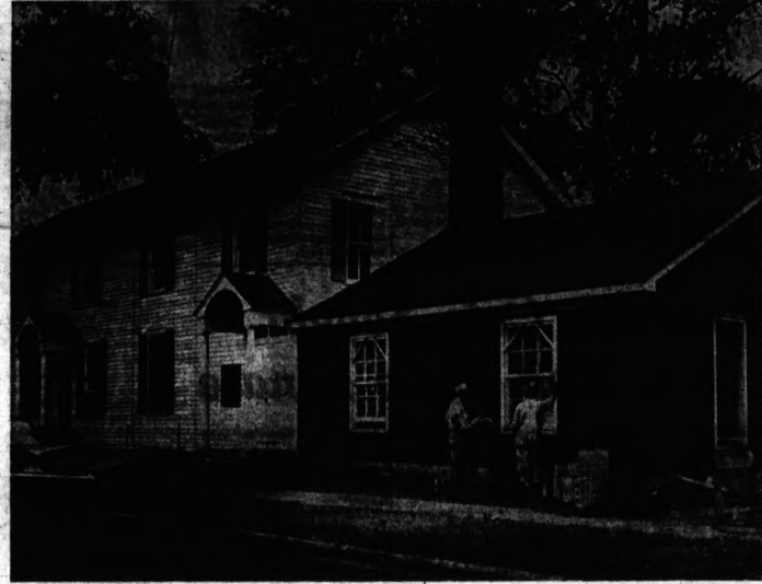
TOWNSHIP HALL ADDITION — Work progresses on the 30-by-30-foot addition to the Avon Township Hall in Rochester, a project finally started last month after some unexpected obstacles were overcome. After the Rochester Zoning Board gave special approval to expansion of the nonconforming use on
