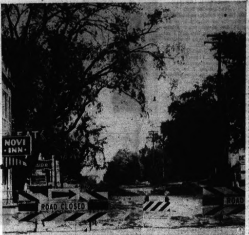
NOVI DETOUR — A $288,000 road rebuilding project on Novi road from Grand River avenue to Eight Mile road will detour traffic from the heavily traveled artery for the next three months, the County Road Commission said today. Replacing the narrow two lane asphalt pavement will be
