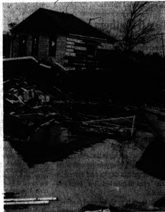
Debris Choked Canal At Anchor Bay
