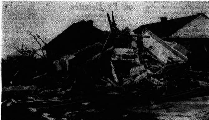
Garages, Houses, Cars — All Reduced To Rubble By Twister's Giant Hand
