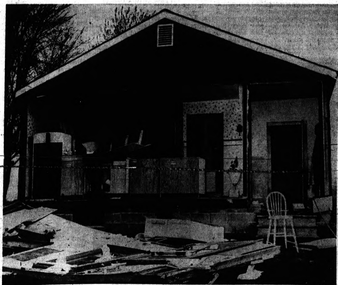
Demon Winds Peeled Off Back Wall Of Lunsford Home On Joslyn
