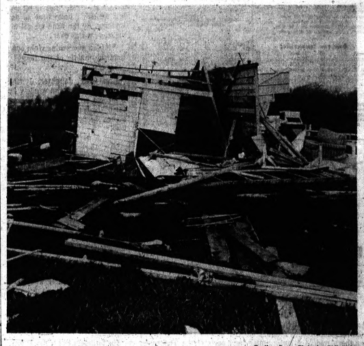
Giddings Road Home Devastated By Tornado
