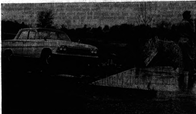
Only Slab Remains Of Richard Lunsford's Missing Garage On Joslyn
