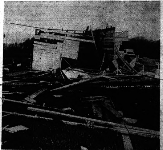
Giddings Road Home Devastated By Tornado
